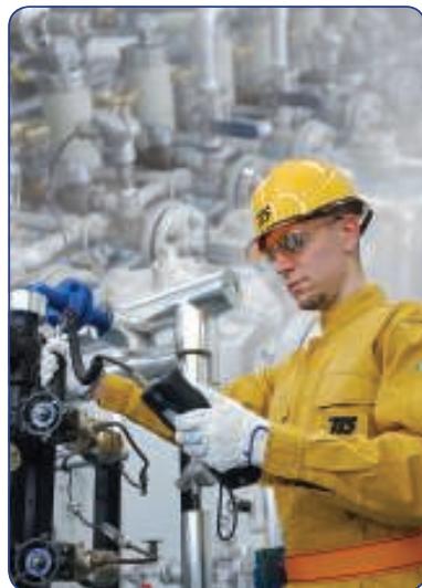
Properly-working steam traps save time and money, and increase safety
