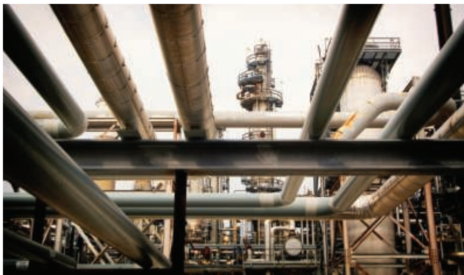
FIGURE 1. Seeing a large CPI facility through design, construction, commissioning and, ultimately, startup requires detailed planning throughout, especially during the project's front end
